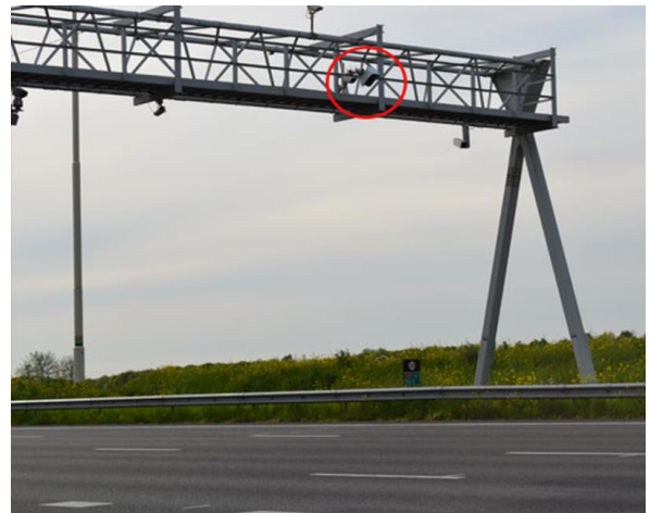
Non Invasive Road Sensor NIRS31 is mounted on a portal above the road
