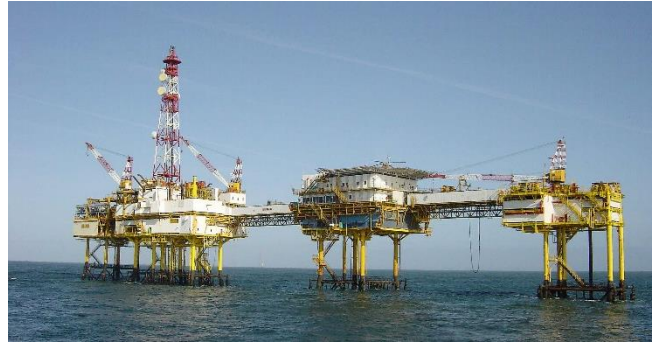
OMC-408 on an offshore platform
